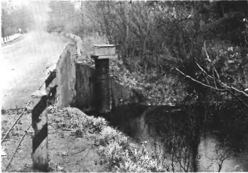
Gaging Station, Mahwah River near Suffern, N. Y.
